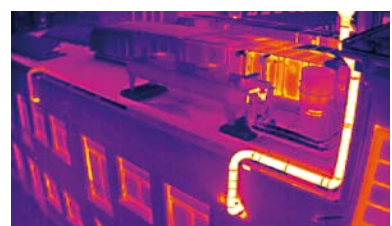
Temperature monitoring for building thermography
